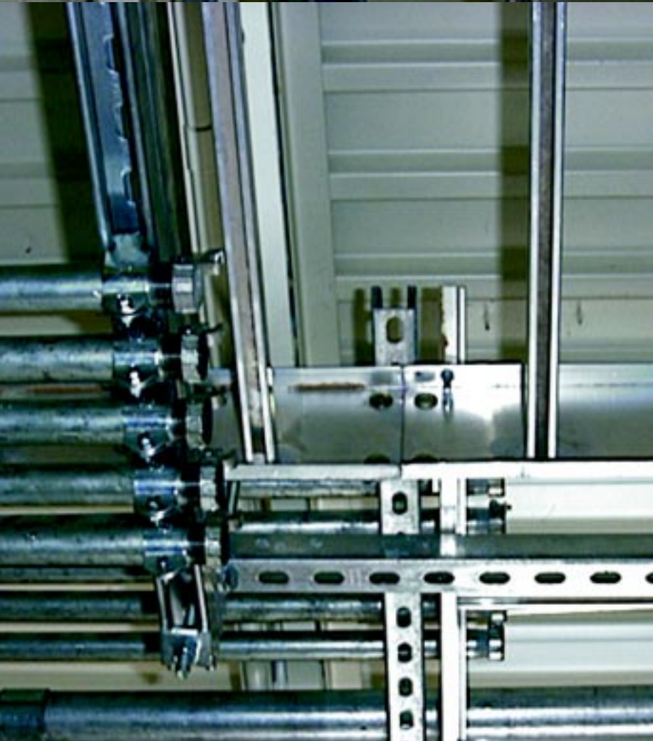
Photo 3 (top) and Photo 4: Ladder-type cable tray and conduit supports at transition points.
